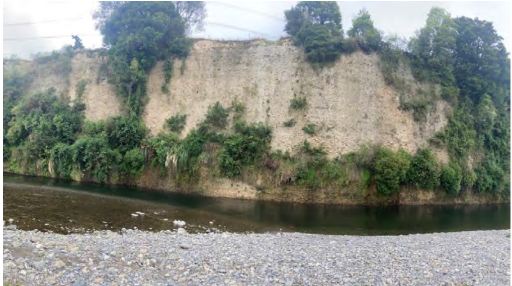
Figure G.19: Potential hydraulic connection between a paleochannel that now forms the water-bearing unit intersected by BH118 and the contemporary channel of the Ohau River, indicated by the line of vegetation 1-2m above the baseflow water level.
